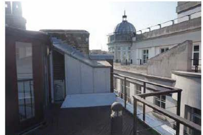
Rooftop looking East view 3
