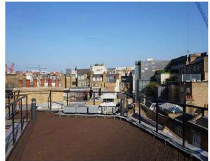
Rooftop looking Northwest
