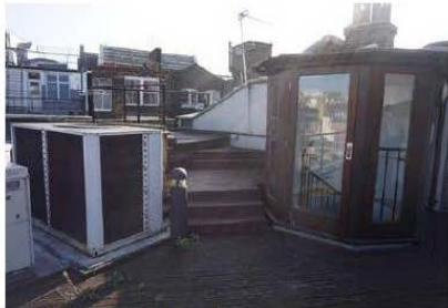
Rooftop looking East view 2
