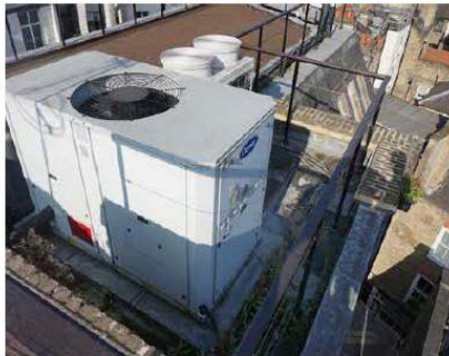
Existing Roof Plant
